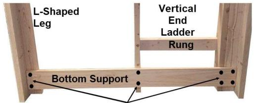
Attach Bottom Support with 1-5/8" screws 1" from the floor to the inside of the legs and back of the Vertical Ladder. Drill pilot holes as needed.
