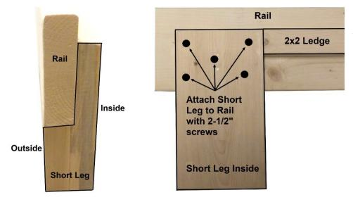
The Short Legs are installed to the inside of the Rail. Depending on the frame height there may be a short board attached to the outside of the leg that the rail will rest on. Attach the Short Leg to the inside of the rail using 2-1/2" screws.
